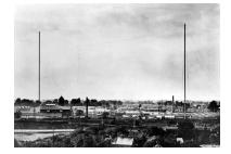
The tall posts in the picture were used to hold up an aerial wire to send radio signals. The aerial had to be high so the radio signal would travel further.
